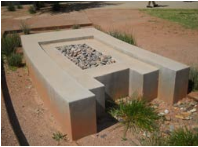
Water features such as the one above can be sustainably designed to incorporate condensate from an adjacent building's HVAC system.
