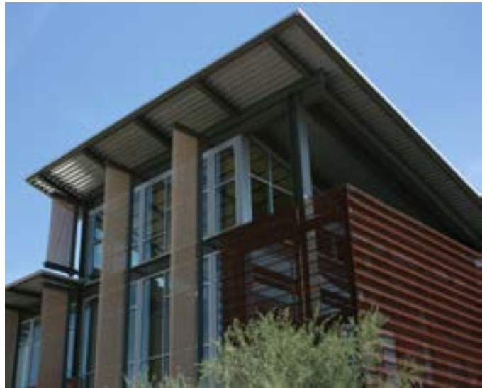
figure 5 - Semi-transparent planar elements serve to establish an architectural rhythm and provide solar control on Picacho Hall.
