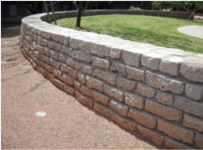
Recycled concrete retaining wall framing the Applied Arts Pavilion amphitheater at the Polytechnic campus.
