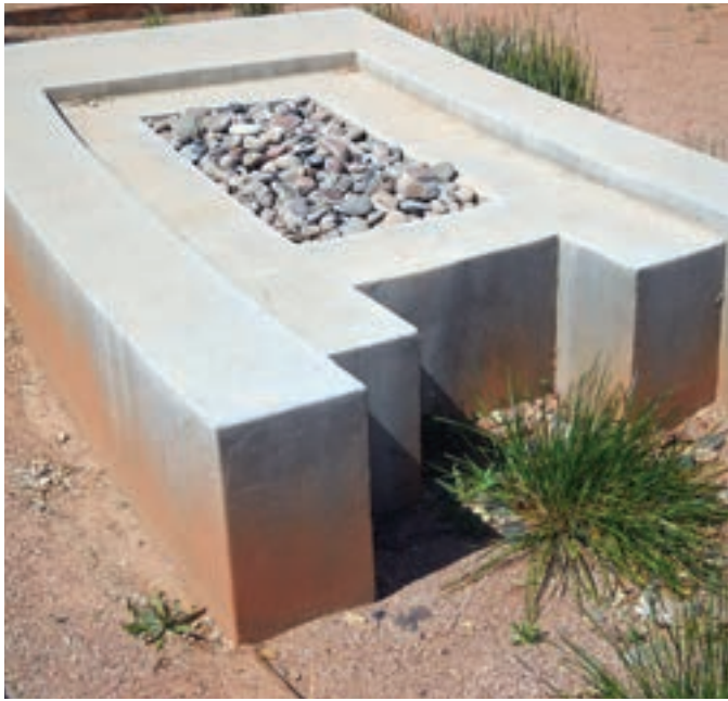
Cast-in-place concrete water features can incorporate building condensate from HVAC systems or be used to showcase irrigation as a water feature.
