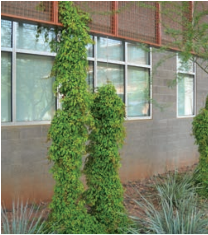
Once established on the metal trellis, this Carolina Creeper vine will help shade and cool the building.
