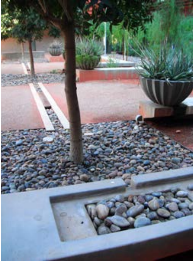
figure 3 - Courtyard at Santan Hall, ASU Polytechnic Campus. Channels in site furnishings and landscape areas direct rainfall to specific trees, expressing and celebrating the hydrology of the site.
