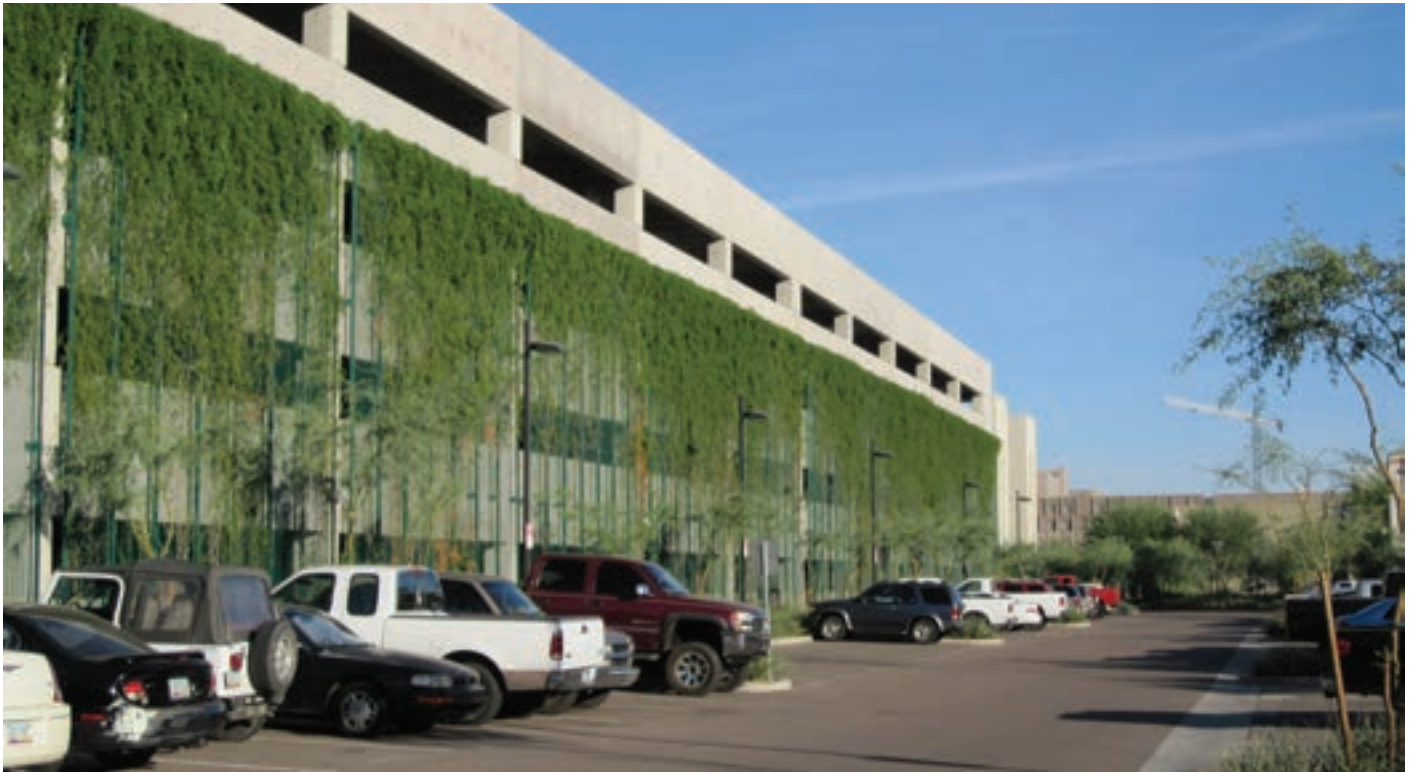
The “green screen” trellis system on this parking structure provides visual mitigation and a reduction in solar heat loading.
