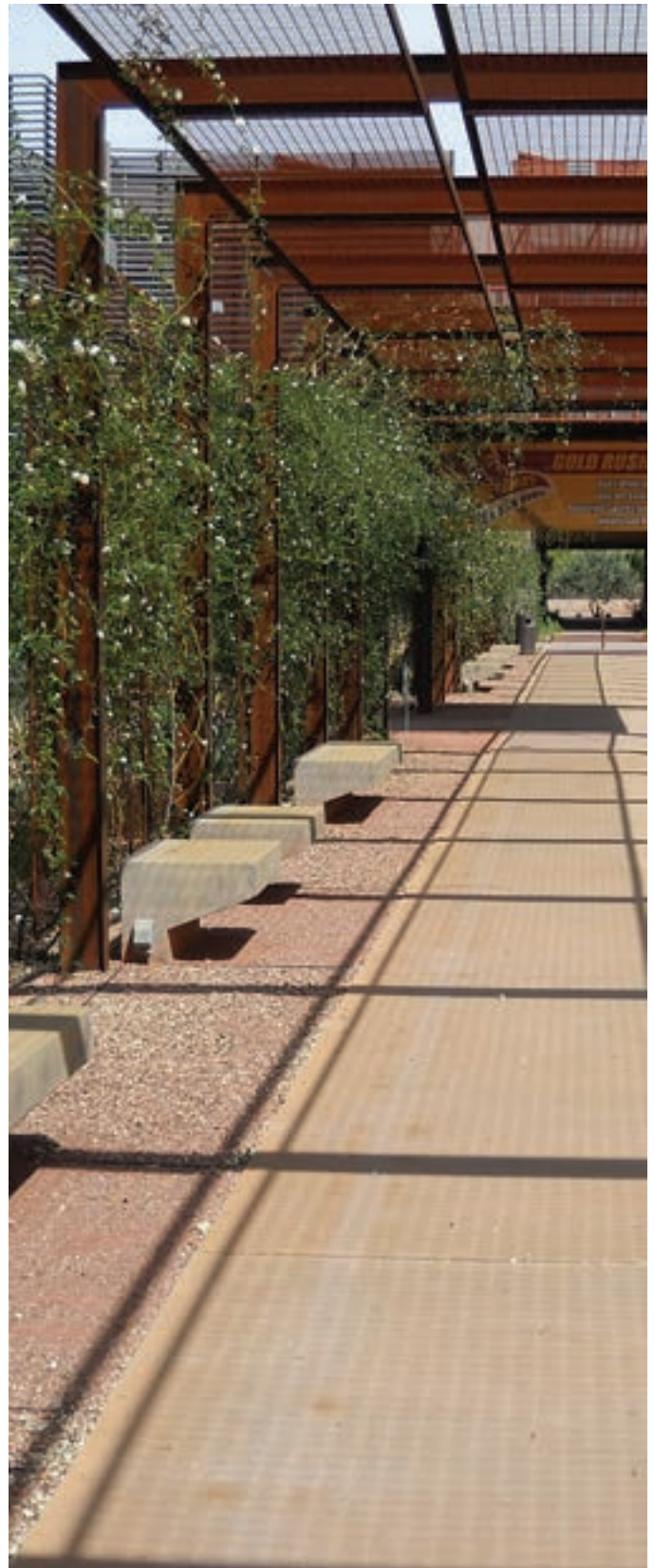
This rusted metal arbor and cast-in-place benches reflect the raw material finishes of the adjacent architecture.
