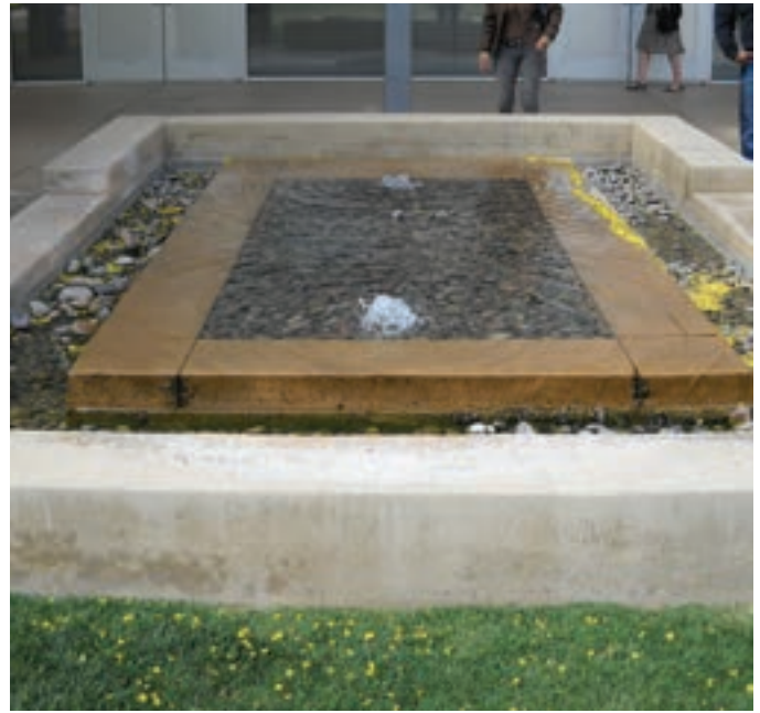
This brimming fountain at the Student Union loses less water to evaporation than typical active fountains.
