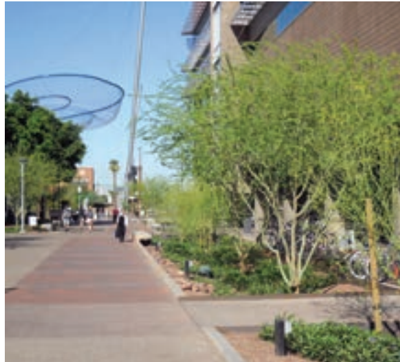
This bioswale benefits from rainwater runoff harvested from the adjacent pedestrian corridor.
