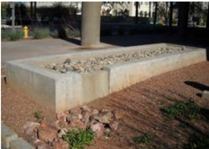
This water feature north of the University Center uses the condensate from adjacent buildings to supplement the landscape irrigation.
