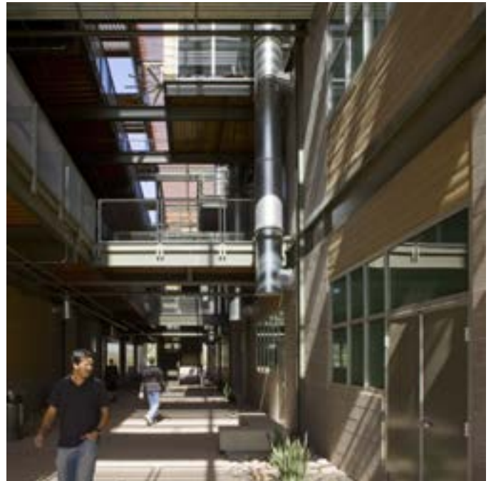
figure 2 - Peralta Hall, ASU Polytechnic Campus. Open hallways pass through buildings creating shaded passages and study spaces.
