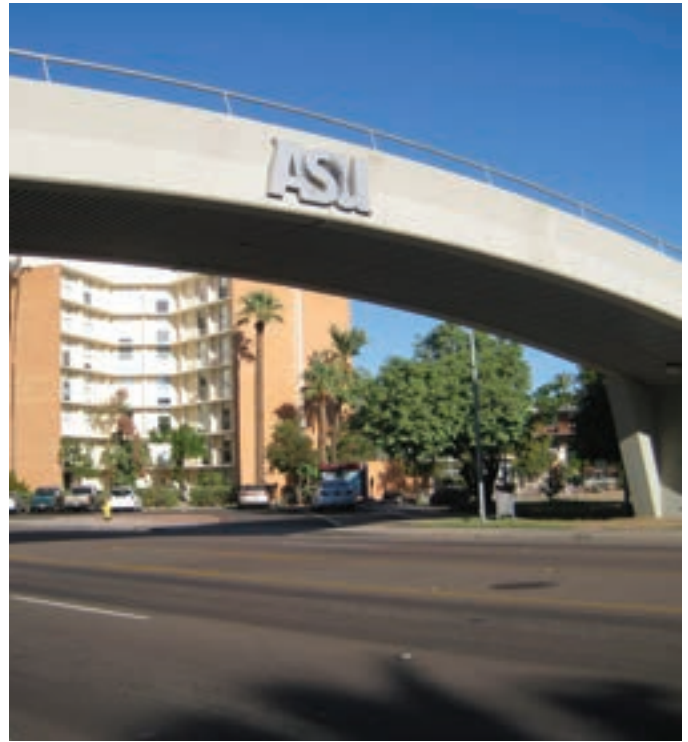
This bridge serves as a gateway and visual indicator to those traveling to the campus.
