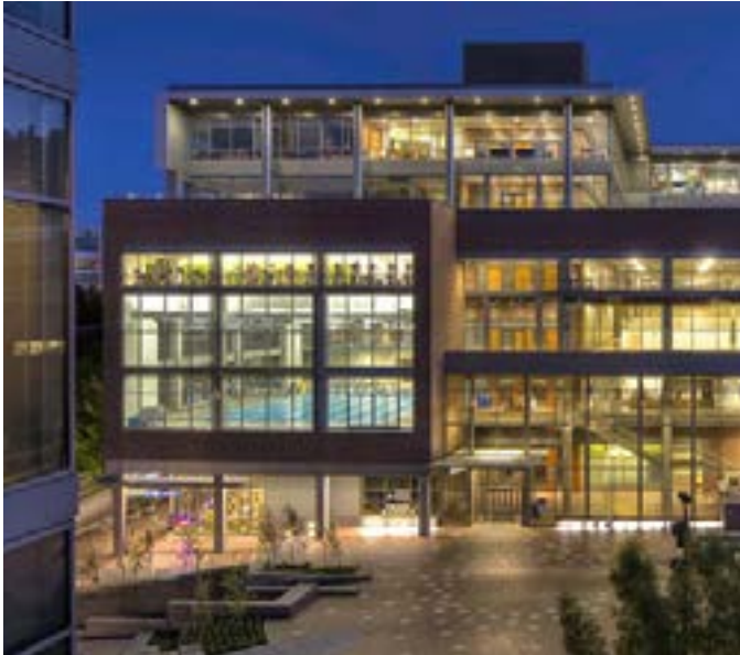
figure 3 - Transparency, program, and site planning make Portland State University's Student Center an active part of the downtown environment.
