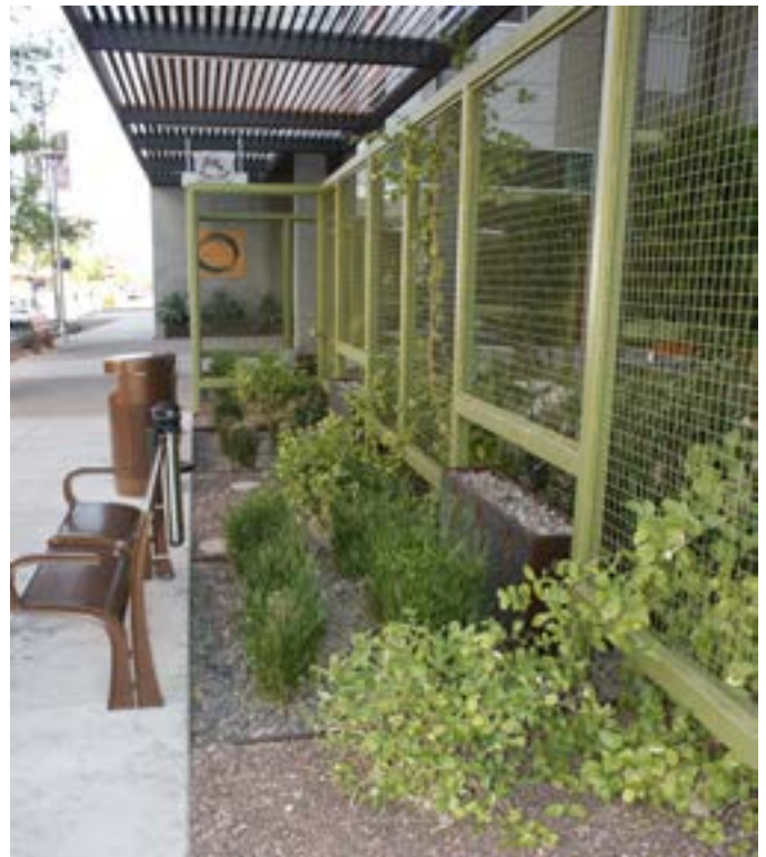
This transitional space takes advantage of vegetative screening to provide shade. The metal trellis is integral to the adjacent architecture.
