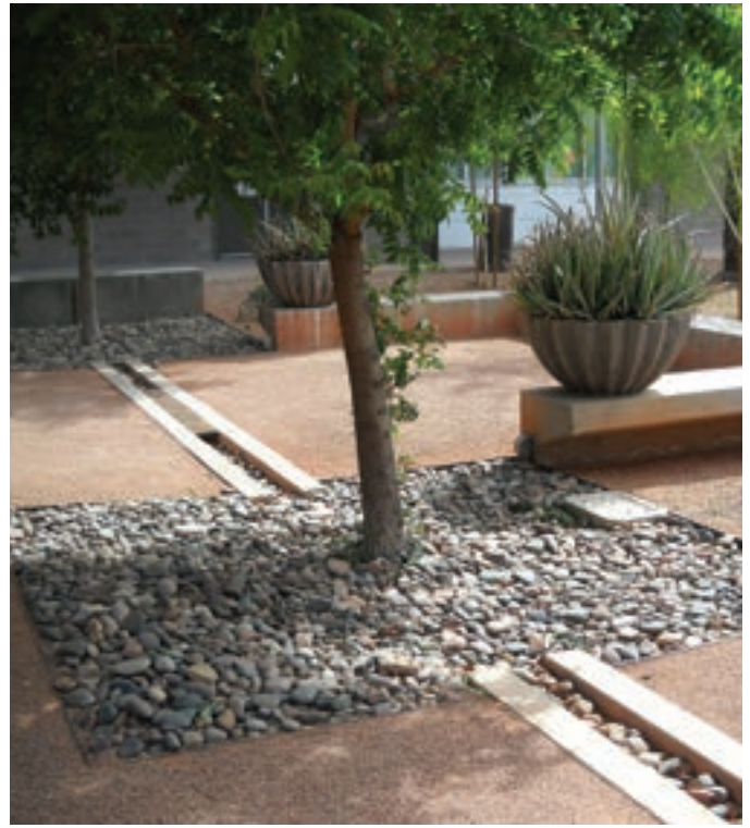
These irrigation runnels direct rainfall and supplemental irrigation to shade trees showcasing the functional relationship of landscape and architecture. .
