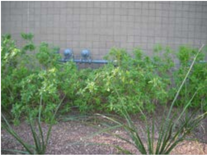
Landscape elements, such as these shrubs on the north side of the Cronkite Building, can be used to successfully screen utilities.
