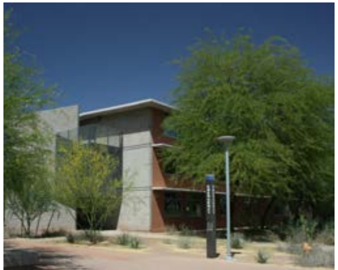
figure 6 - A stairway addition to Wanner Residence Hall creates a distinctly contemporary wing while relating to the original construction.
