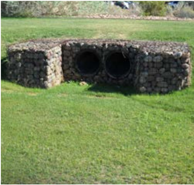
Normally mundane site infrastructure such as storm drain headwalls can be designed in such a way as to contribute to the cohesive campus identity.
