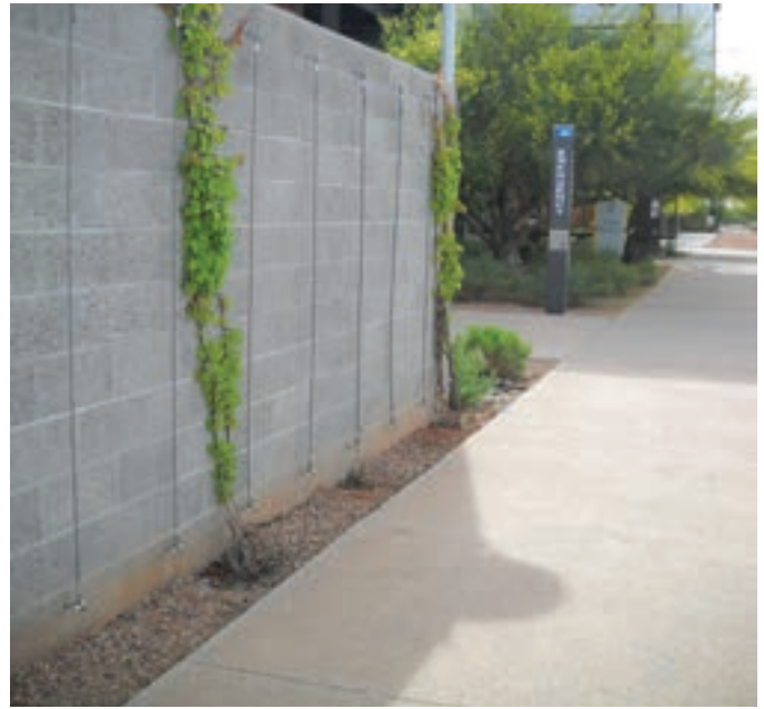
This cable trellis system and creeping vine will provide a “green screen” that will reduce solar heat loading as well as screen unsightly utilities.
