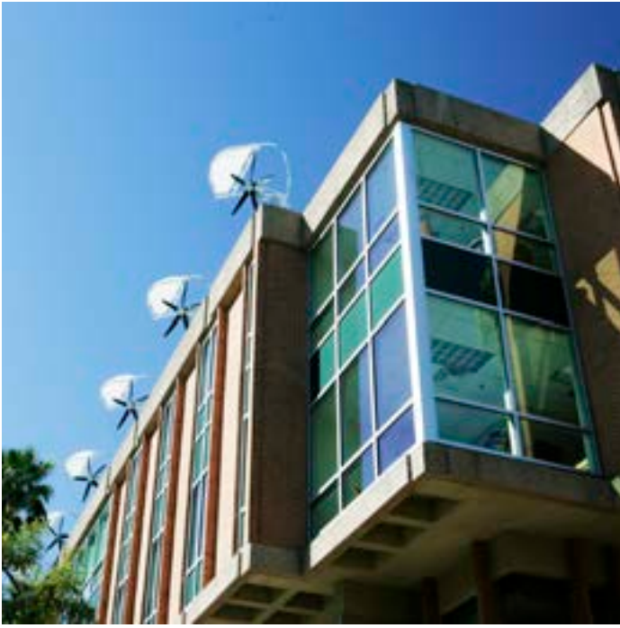
Wind turbines on the Global Institute of Sustainability building.
