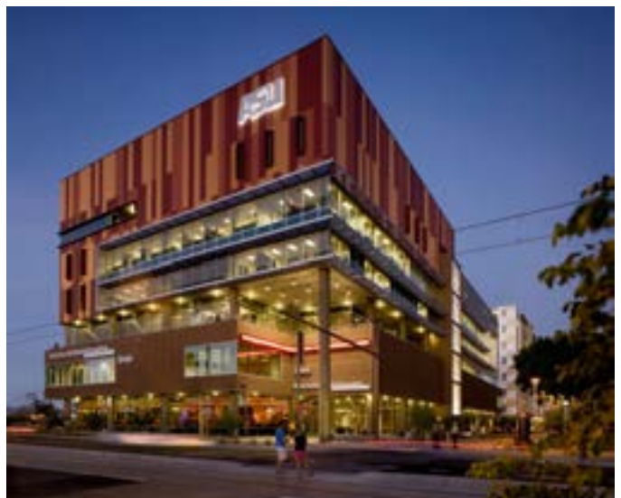
figure 2 - The Walter Cronkite School of Journalism and Mass Communication, ASU Downtown Campus. Building massing and materiality reduces the scale of a large volume, creating a more pedestrian volume on the lower floors with transparency along the street edge.
