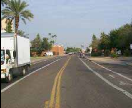
McAllister Avenue - Two Way Traffic - Bicycle Lane
