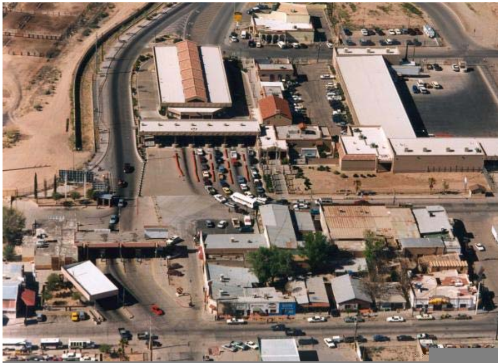
Picture 1: Diagram of the Douglas Port of Entry into the United States. Commercial vehicles enter into the docking bay on the far right, while passenger vehicles use the five passenger lanes to the left. Source: Border Infrastructure Project, http://www.bip.arizona.edu/
